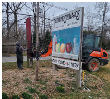
Fence post pounding: Installing new fence at the main farm
